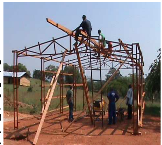
Erection of Beekeeping Project workshop
